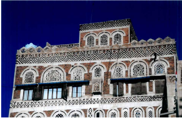
A house of Sana'a showing the belt (az-zinnar) between floors
