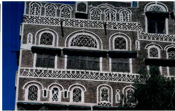
Shutters for the wooden windows of
